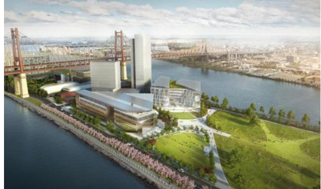
Fig. 3 Areal view of the new Cornell Tech Campus, Roosevelt Island, New York.
